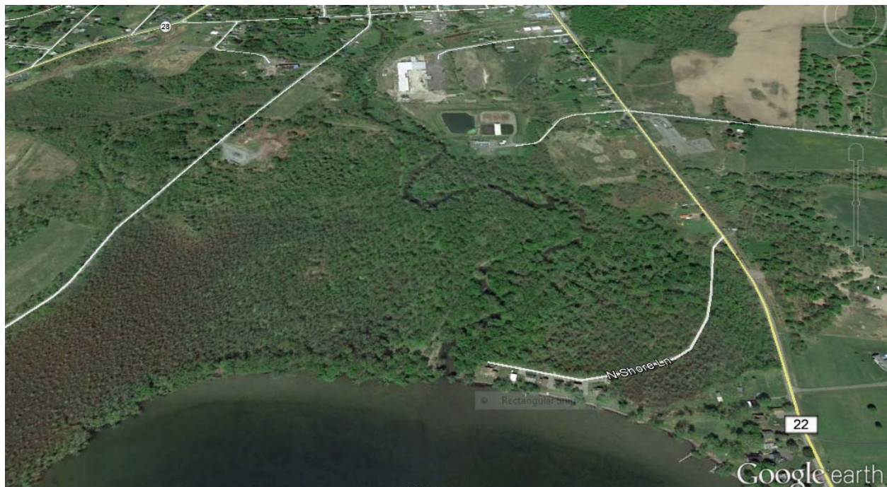
Figure 14: A new beach? The north end of Canadarago Lake and Richfield Springs beyond.
